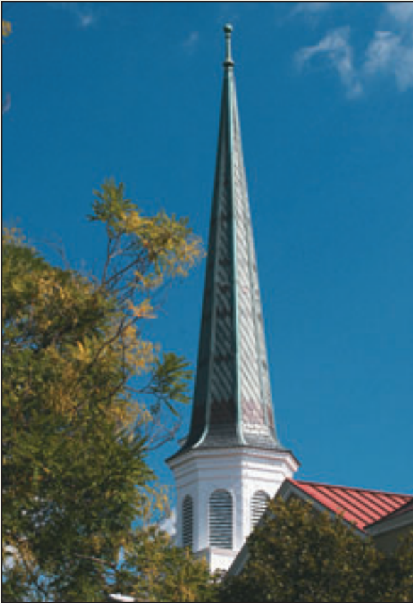
Downtown Baptist Church , 212 S. Washington Street, Alexandria, VA. Originally built in 1803, the steeple was added in 1858. New Buckingham slate and copper hip metal. Base of steeple restored and painted.
