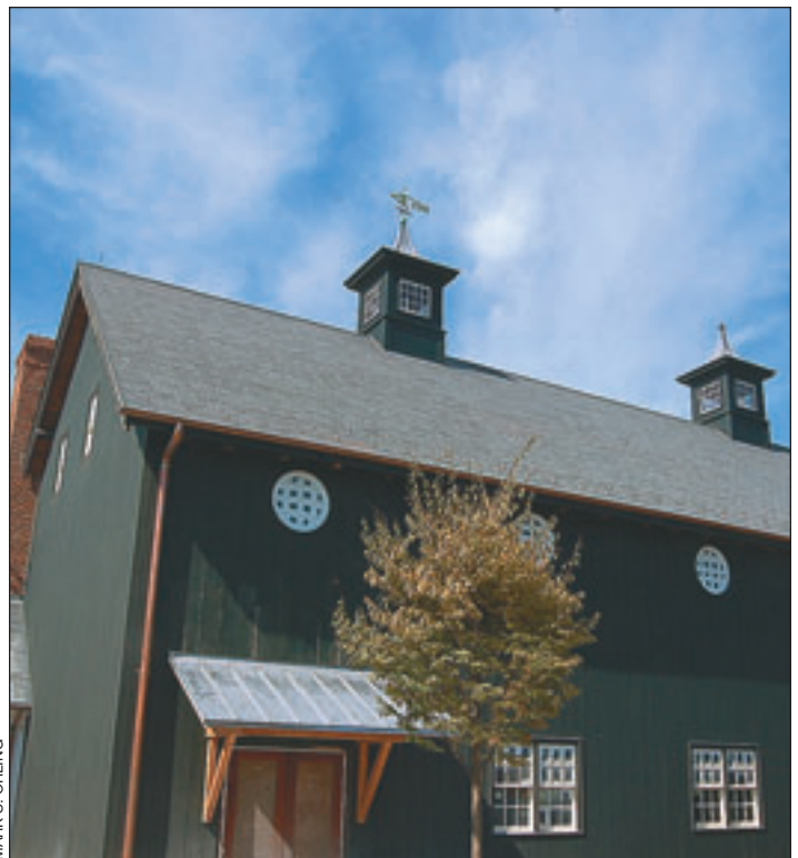
Wagner Roofing installed synthetic slate on the Chandler Barn (c. 1855).
