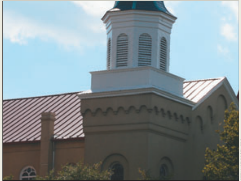
Downtown Baptist Church , 212 S. Washington Street, Alexandria, VA. Originally built in 1803, the steeple was added in 1858. New Buckingham slate and copper hip metal. Base of steeple restored and painted.
