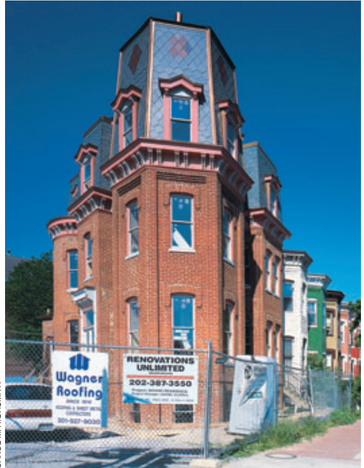
Working from photographs and a home video, Wagner replicated the hand-cut slate roof on this 1878 home.
