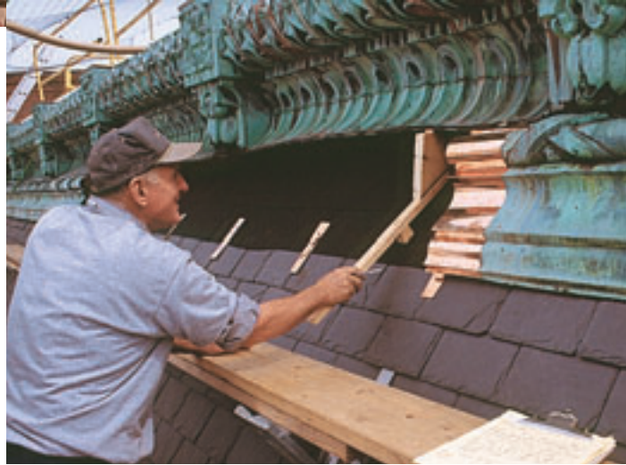
(Left) Tony Tejada installs new pressure-treated plywood to replace the failed concrete deck. The Old Executive Office Building and American Red Cross headquarters can be seen at upper left. (Below) Bob Wooldridge rebuilds the structure that supports the Folger's restored copper cornice.
