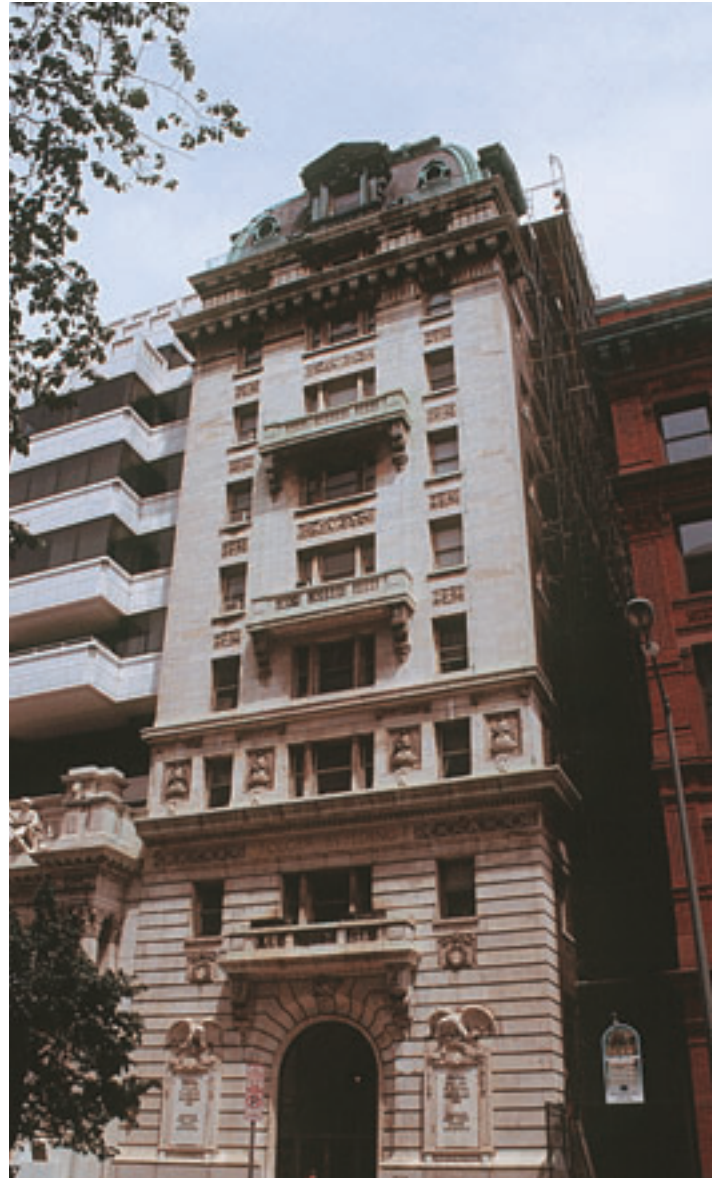
Wagner is restoring the Folger's 1907 exterior.
