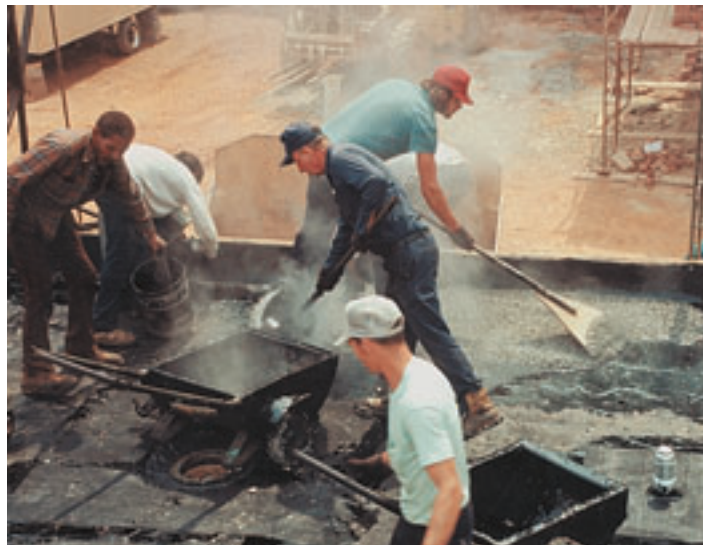
Early Jones (center) leading his built-up-roof crew.
