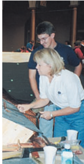
(Above) Jeff Wooldridge demonstrates slate repair. (Right) Sheila Wagner uses a "ripper" to remove a broken slate.
