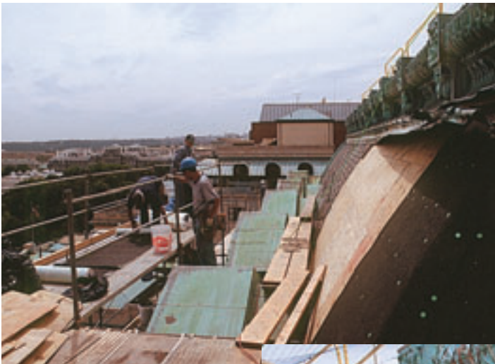
(Left) Tony Tejada installs new pressure-treated plywood to replace the failed concrete deck. The Old Executive Office Building and American Red Cross headquarters can be seen at upper left. (Below) Bob Wooldridge rebuilds the structure that supports the Folger's restored copper cornice.
