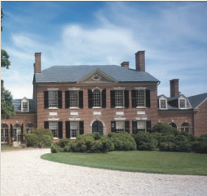
Woodlawn Plantation , 9000 Richmond Highway, Alexandria, VA. Buckingham slate, copper roofing and gutters and downspouts.
