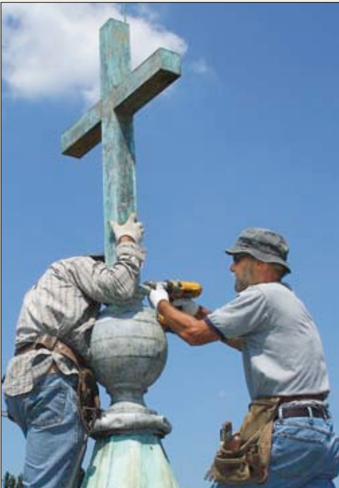
St. Paul's Episcopal Church (Built in 1719) , Rock Creek Church Road & Webster Street, NW, Washington, DC. New slate roof, copper built-in gutter, copper roofing on the steeple, copper cross painting and restoration.
