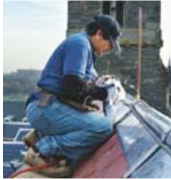
Jose Santos installs lightning rods and lead-coated copper ridge cap.
